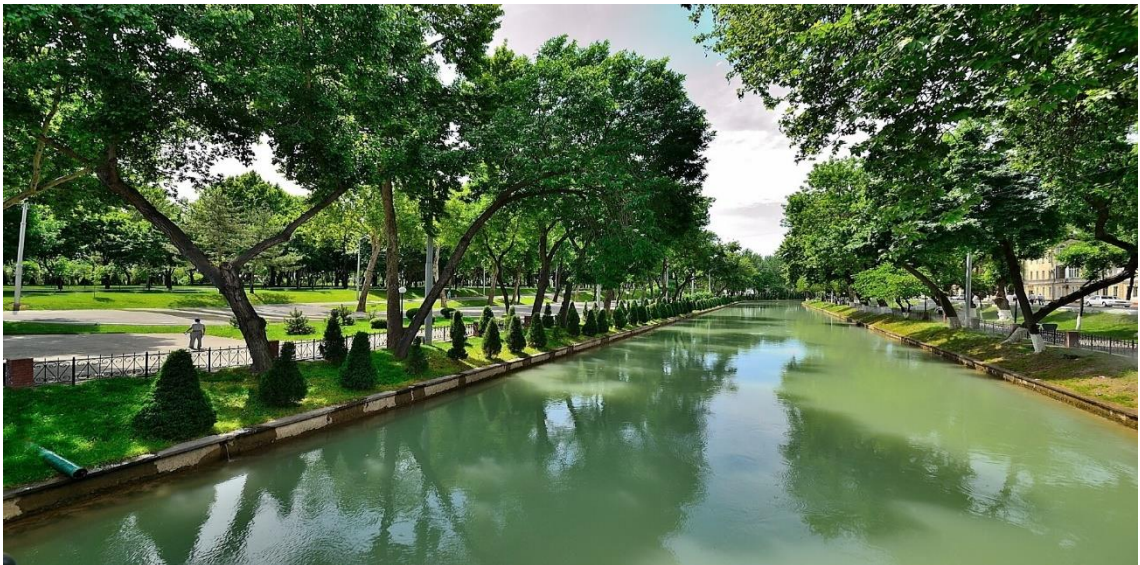
Fig.1. Ankhor Canal embankment
