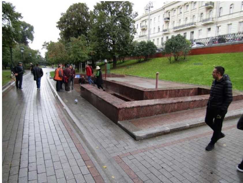
Fig.7. Underground public toilet
